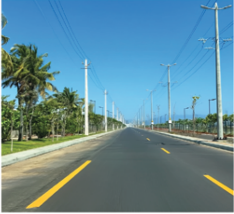
Entrance - Sector 2A
