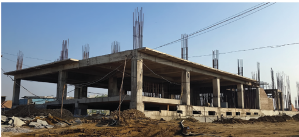
120-Bed Hospital (in Phase 1)
